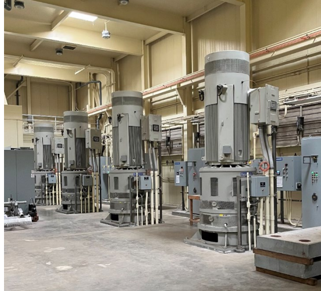
Four Dynamatic 450 hp 514 rpm vertical eddy current drives.
